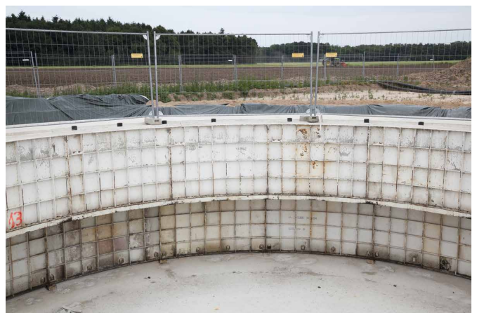
WEA4 / Innenhohlraum Fundament
