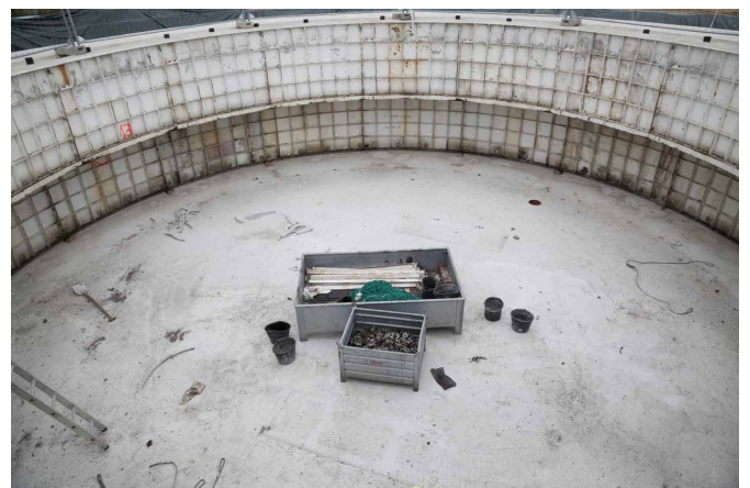
WEA4 / Innenhohlraum Fundament
